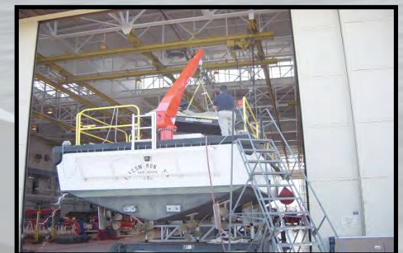
Target Boat Boom Crane Test
