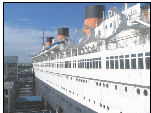
Queen Mary Port Side View Looking Forward
